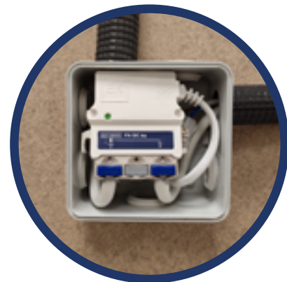
80x 80 mm junction box installation
